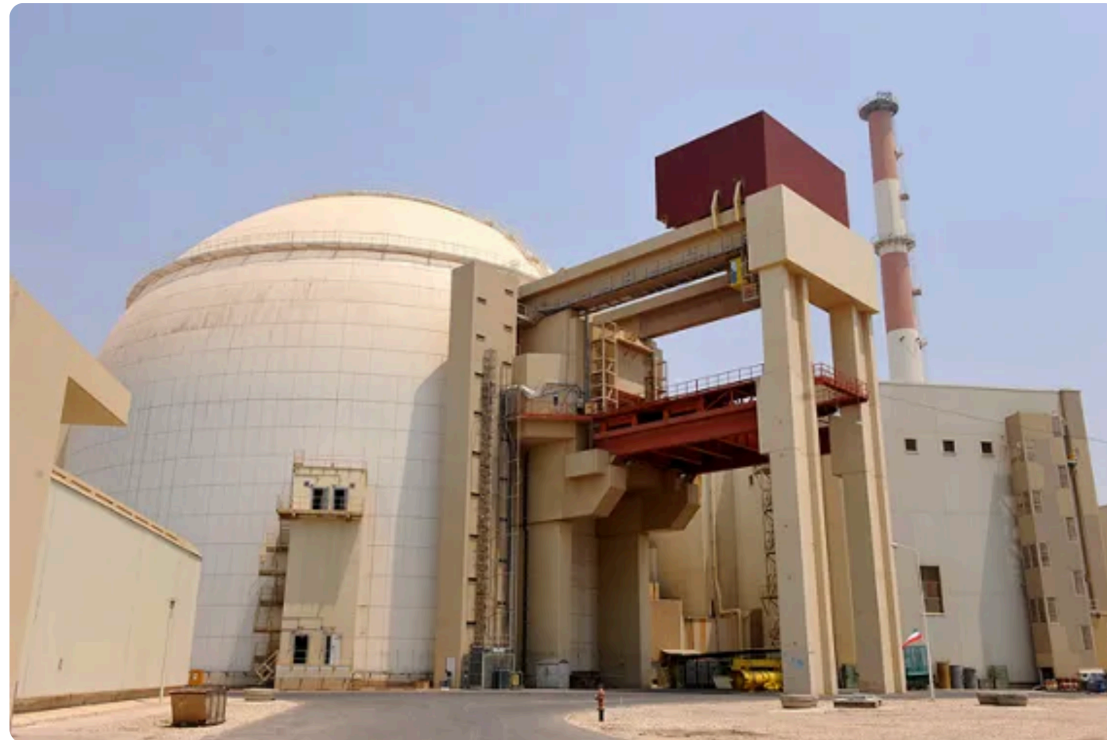
The reactor building at the Russian-built Bushehr Nuclear Power Plant as the first fuel is loaded, on August 21, 2010 in Bushehr, southern Iran [IIPA via Getty Images]
